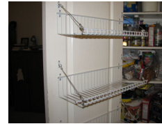
Upper shelves installed- shorter for clearance!
